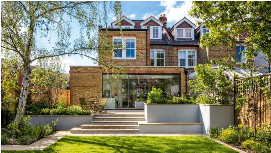
Figure 3: Contemporary/contrasting extension on a traditional style house built using matching brick with quoins, heads and banding detail to match the existing dwelling (Image credit: Grant Architecture and Interiors)
